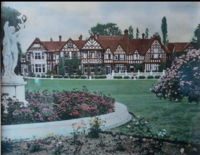
The present marble shown in situ at The Willows, Windsor, England, early 20th century.
